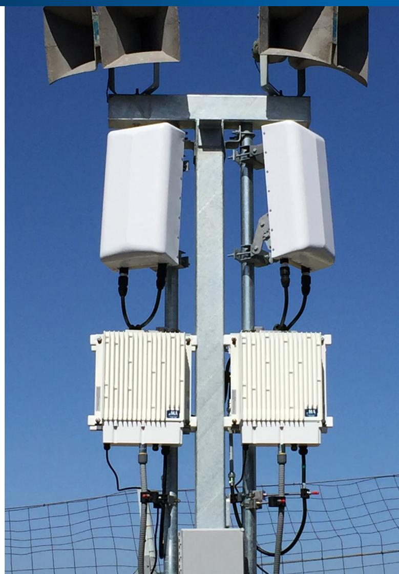
**FUZE provides digital electricity to antennas and remote units deployed in the far reaches of the raceway.**
